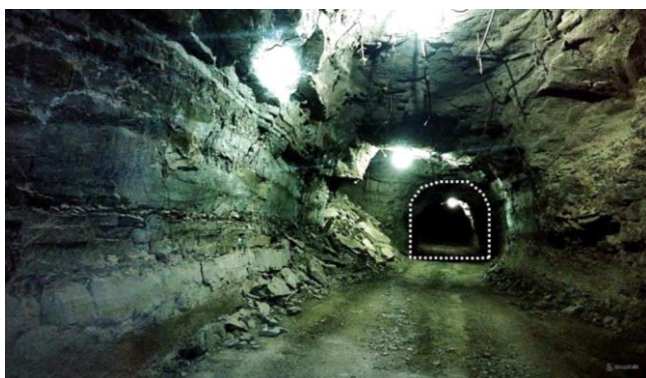
Figure 2. Destruction of the haulage drift 1 wall from the side of panel 7
